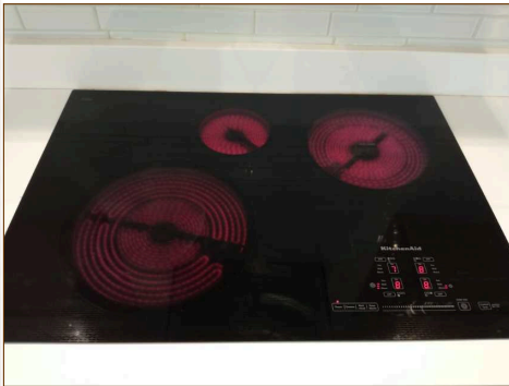
All burners appear operational
