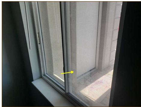
Seal failure
