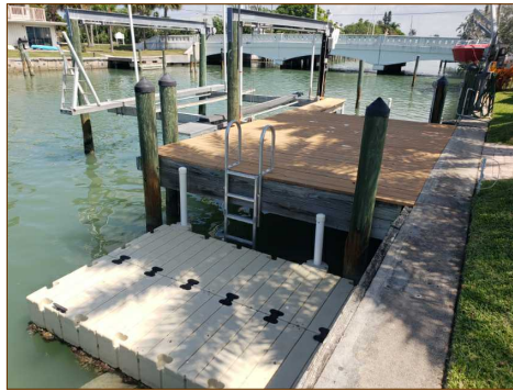
Wood pilings and wood/trex decking
