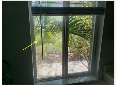
Seal failure
