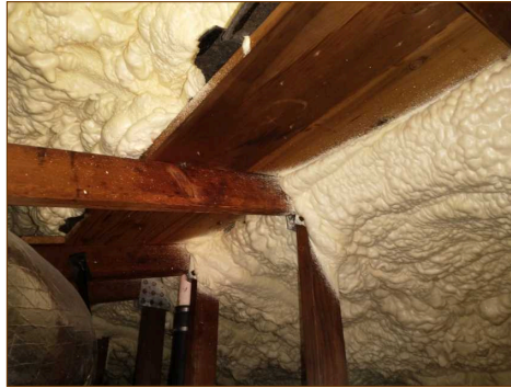
Dimensional lumber sheathing, Some plywood likely
