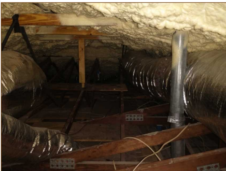
Truss framing, sheathing not visible
