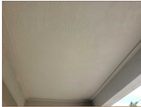
View of front patio ceiling
