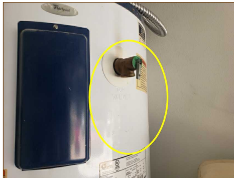
Extended TPR drain line as needed
