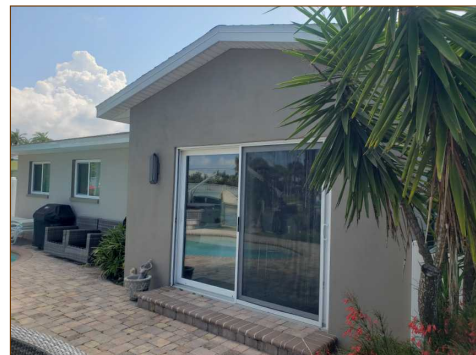
View of rear patio area
