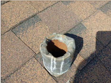
Cast iron waste lines
