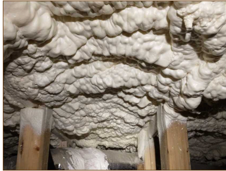
About 4 inches thick for an R-value of R-38.
