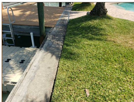
Seawall backfill is adequate
