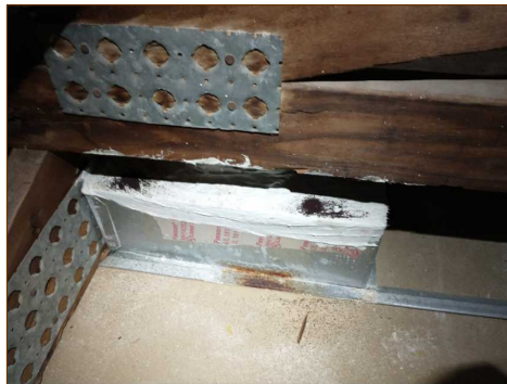
Past wood eating insect activity suspected
