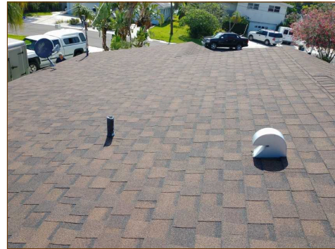
View of flashings
