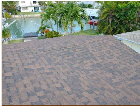
No ridge ventilation, sealed system
