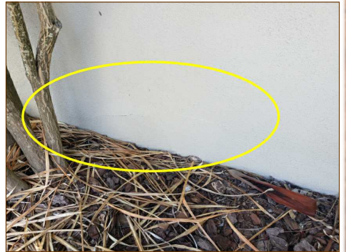
A bit more than typical cracked stucco. It's loose.
