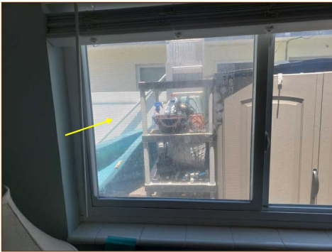
Seal failure
