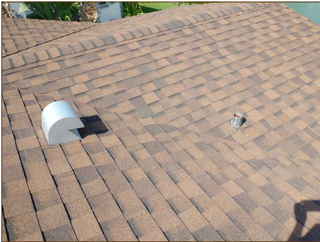
View of flashings
