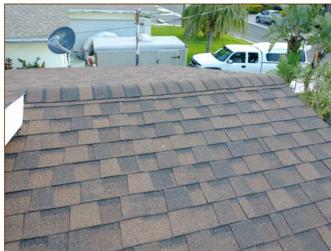
No ridge ventilation, sealed system
