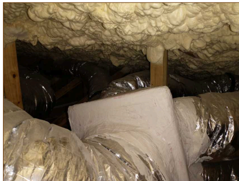
No supply ductwork in attic space
