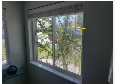
Seal failure
