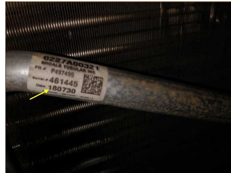
Coil looks to have been replaced in 2018
