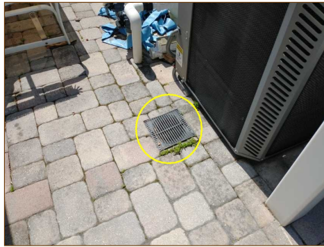
Subsurface drain(s) noted
