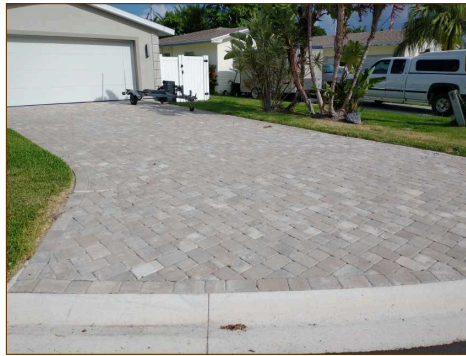
View of driveway
