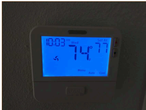
Set up to allow home to equalize and inspect A/C unit
